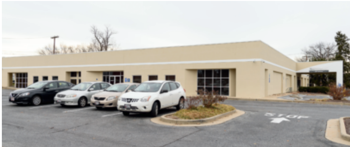
FMH Toll House at 501 West 7 th Street. For best access to the building, use the Toll House Avenue entrance.
